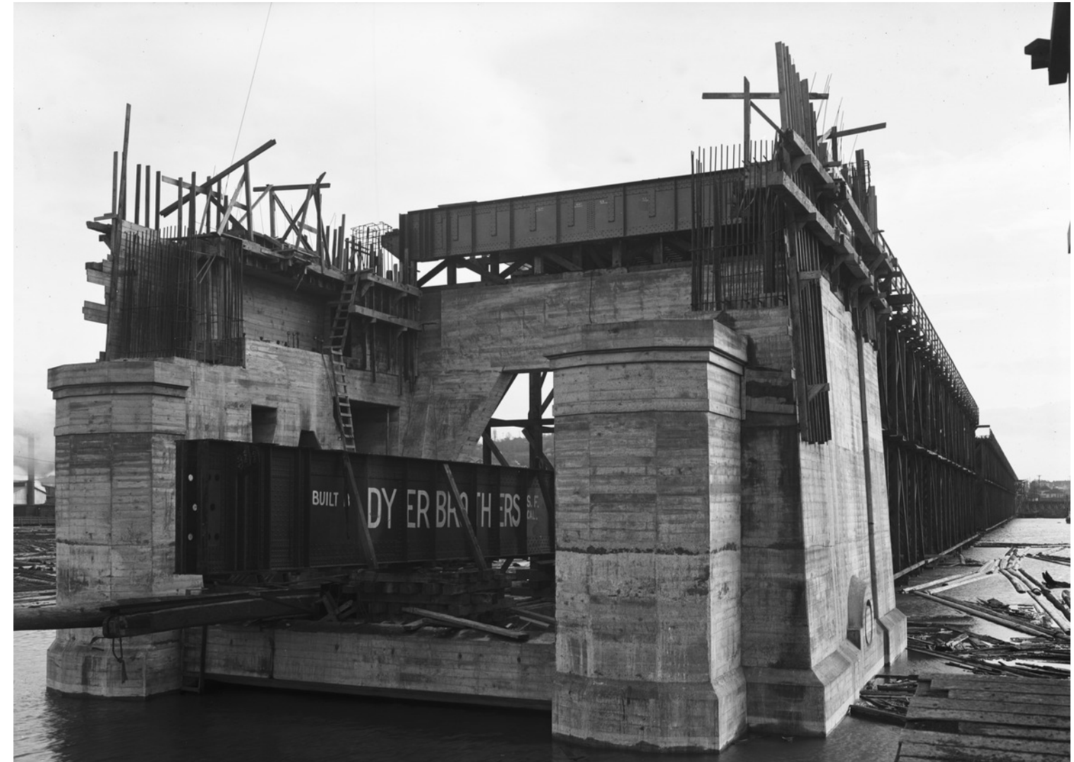
Ballard Bridge under construction in 1916
